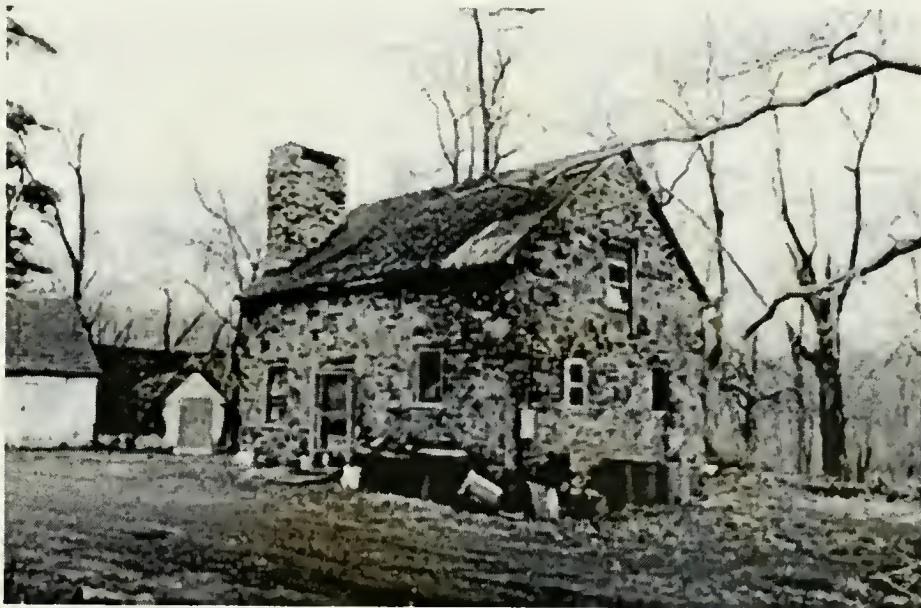
Figure 28 Caretaker’s Cottage, looking southwest, 2001
